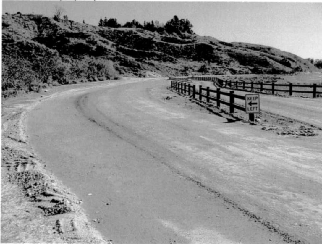
10. South of wetlands, looking east, showing possible encroachment of County Flood Control road on easement property:
